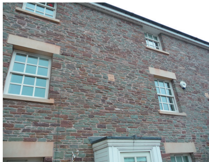
Fig 3. Red and green sandstones in new build in Hay-on-Wye.
