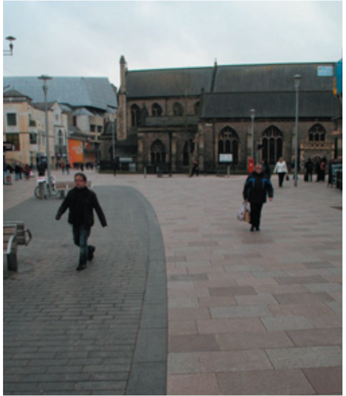
Fig 3b. Granite and olivine gabbro paving, north end of St. John's Street/Working Street, Cardiff.
