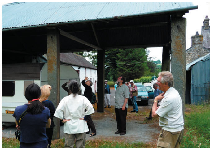
Fig 5. Long columns of Llandewi Brefi Bluestone supporting the barn roof.
