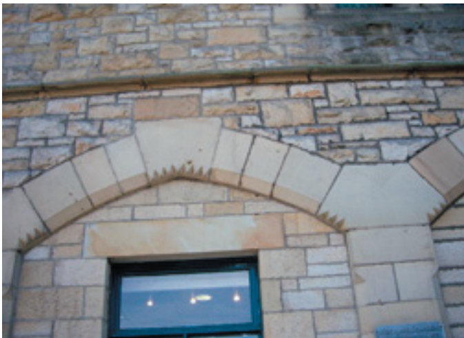
Fig 1. In-filled arches of the Town Hall.
