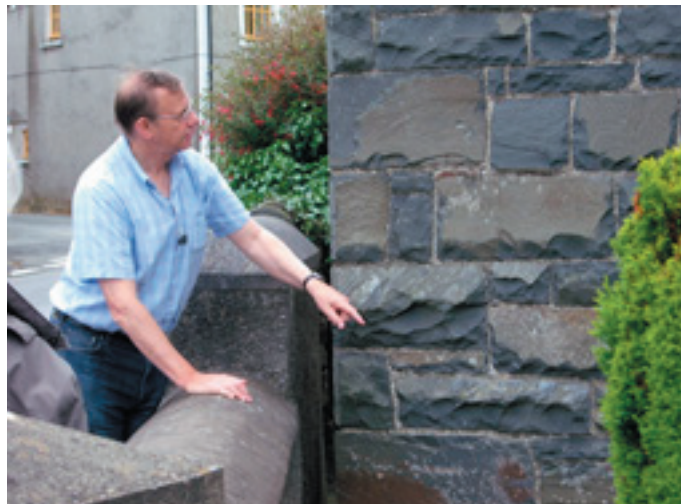
Fig 4. Tim Palmer examining the walls of a house constructed of Llandewi Brefi Bluestone.
