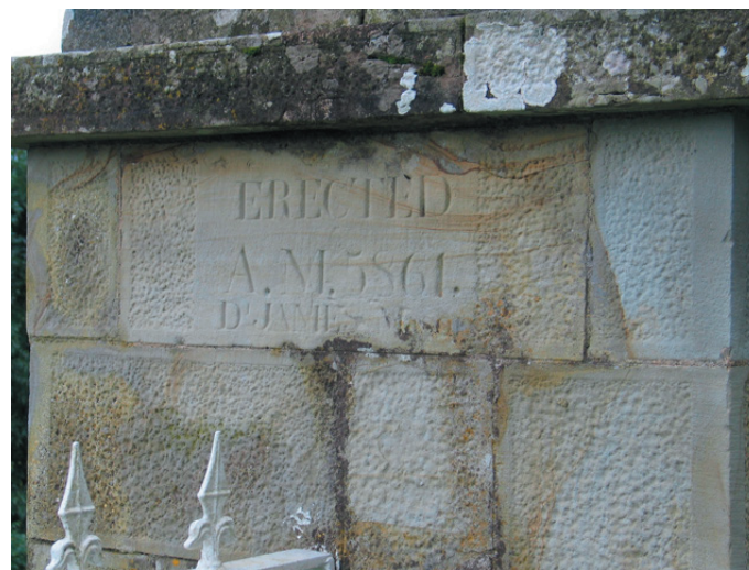
Fig. 3. Gatepost at Bwlchbychan House giving building date as Anno Mundi 5861.
