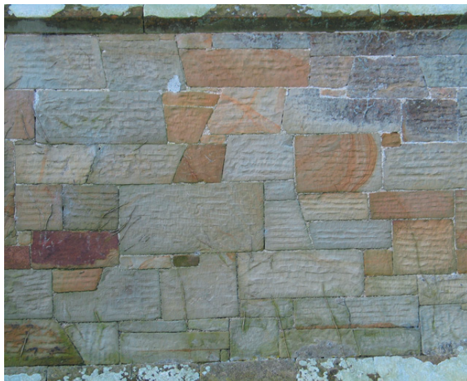
Fig. 1. Pwntan Stone, lower exterior of east end of Tremain Church.
