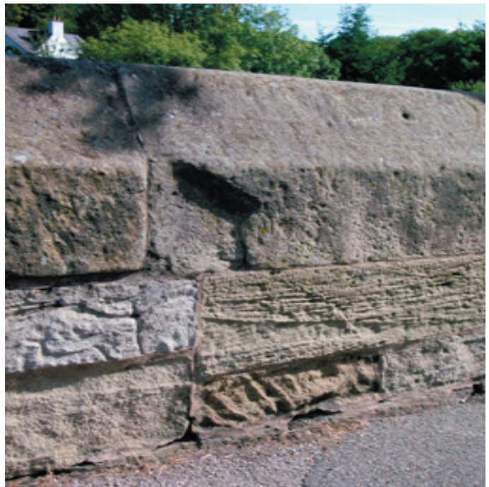
Fig 3. Cefn Sandstone coping stones on the old bridge, Llangollen.
