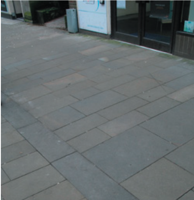
Fig 1. Forest Pennant paving Park Place, Cardiff.
