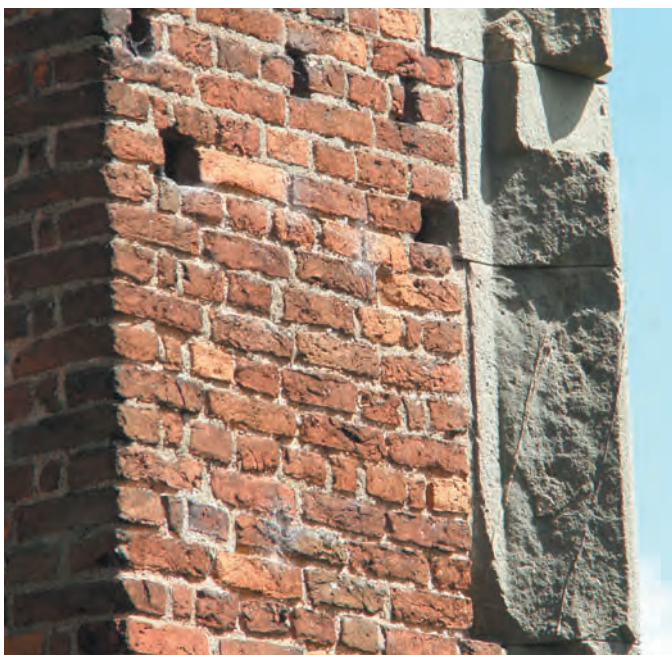
Fig 4. Morton Corbet Castle. Elizabethan outer skin of Grinshill stone with load-bearing brick structure behind.
