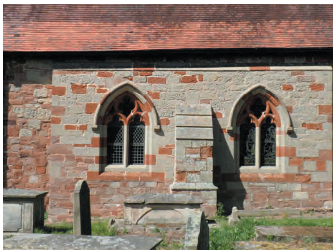
Fig 6. St Andrew, Stanton-upon-Hine Heath. Close up of patchwork white and red Grinshill Sandstone in buttress.
