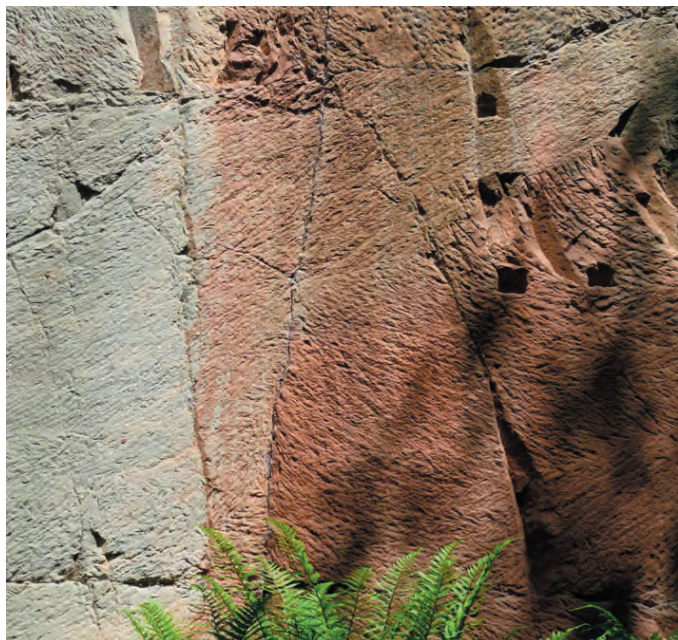
Fig 2. Bridge Quarry showing numerous tool marks in the sandstone. Note also the variation in colour of the sandstone produced by removal of iron.
