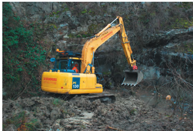
Fig 2. Conservation work clearing exposures of Newmead Sandstone.
