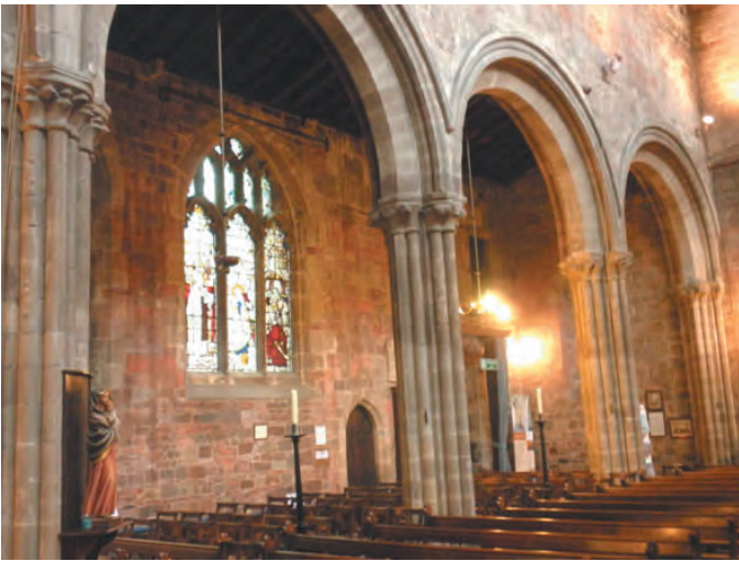
Fig 16. St Mary's Church, Shrewsbury, with contrasting stone in the walling and arcade.
