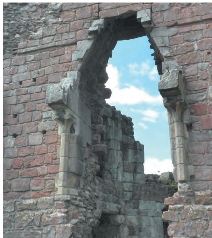
Fig 3. Morton Corbet Castle, thin pink Grinshill Sandstone facing with rubble stone behind.
