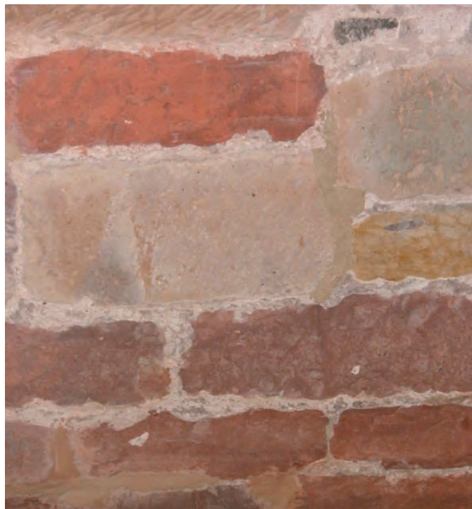
Fig 15. Internal wall of Old Shrewsbury School showing construction from rough coursed local stone.
