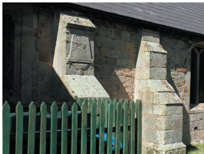
Fig 7. St Mary's church, Shawbury. Buttress with part of a reused or unfinished gravestone.
