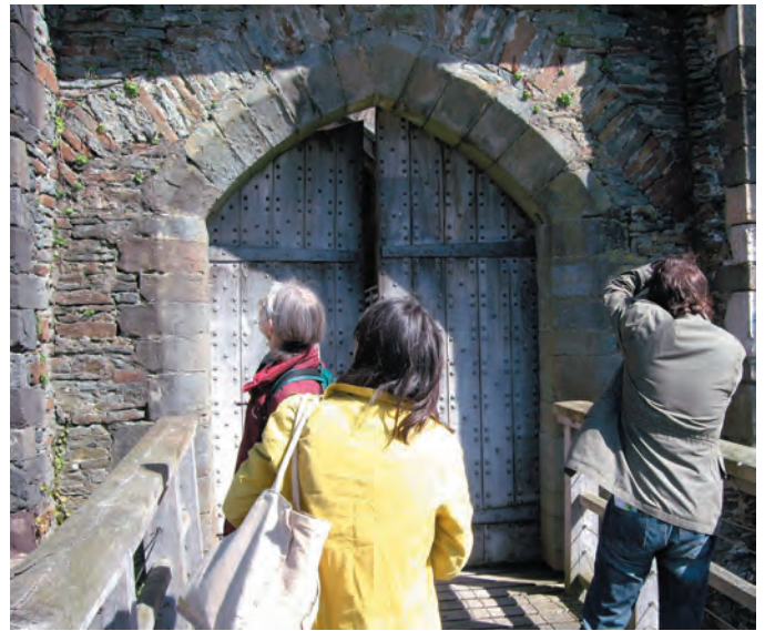
Fig 2. The west gate
