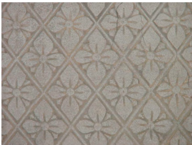
Fig 17. Example of moulded plasterwork, St Mary's Church, Shrewsbury
