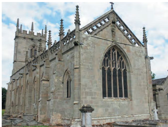
Fig 8. St Mary Magdalene, Battlefield. Eroded patches of stonework, view north.
