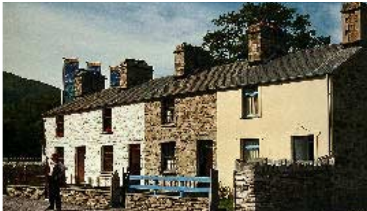
The Fron Haul row of quarrymen's houses at the Welsh Slate Museum, Llanberis.
