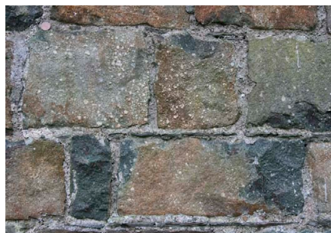
Fig. 1 (top). Cana Independent Chapel, Felindre Farchog. Fig 2 (bottom). Squared, hammer-dressed blocks of ‘spotted’ dolerite forming Cana’s façade. The penny-piece, top left, is for scale.
