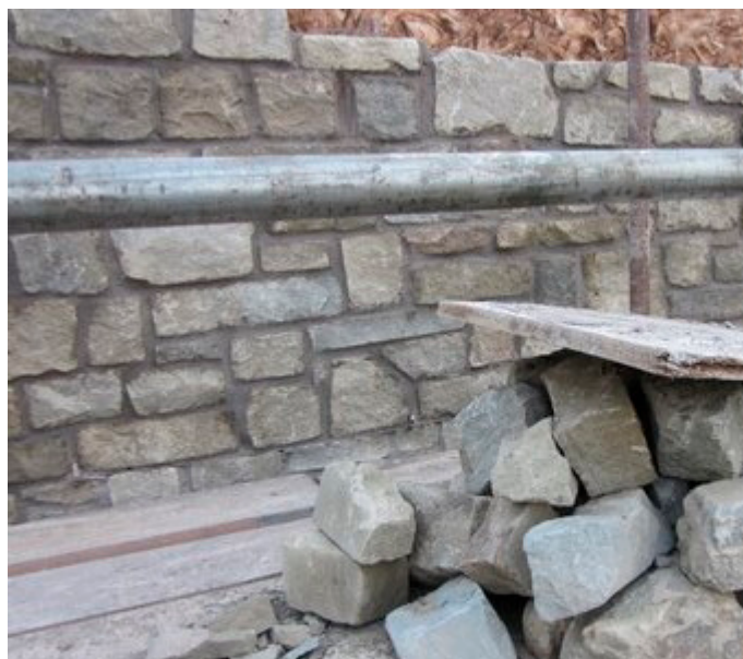
Fig. 2. Uncoursed stone work in new build.
