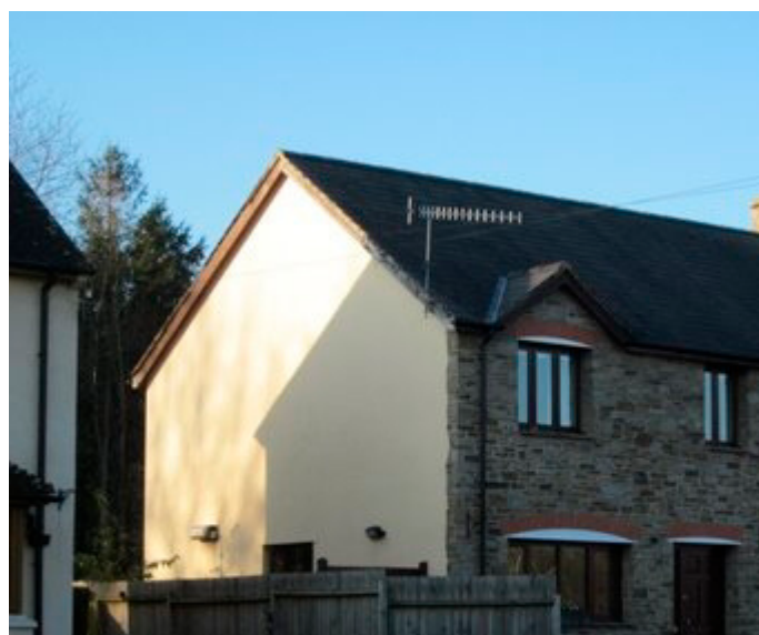
Fig. 1. Typical stone front-faced new build.
