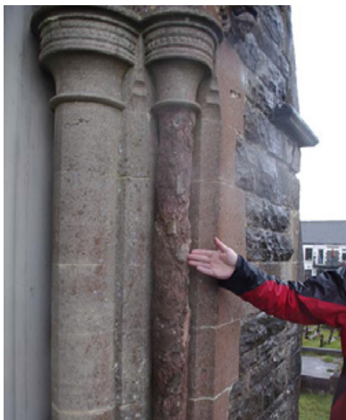
Fig.2. Weathered columns of Radyr Stone, St Augustine's Church, Penarth
