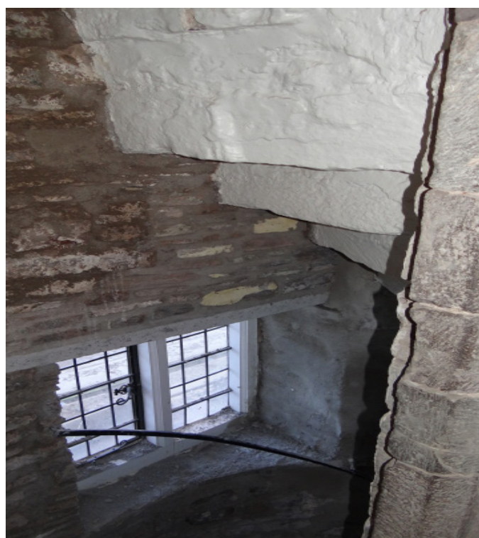
Fig. 6. (Top left). Bricks inserted into the existing masonry during Caroë's renovation.
