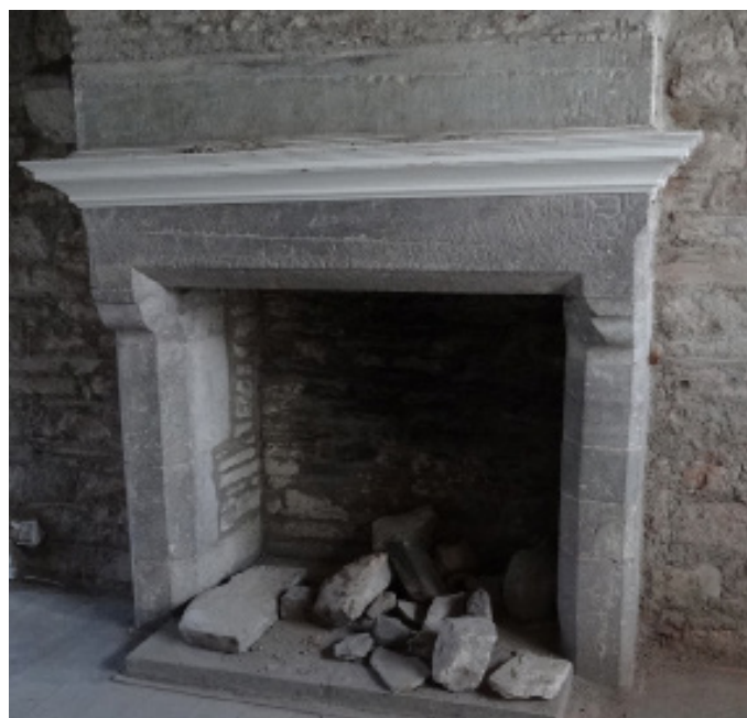
Fig. 6. (Top left). Bricks inserted into the existing masonry during Caroë's renovation.
