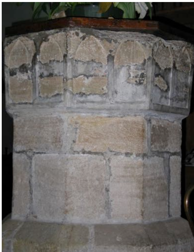
Fig. 2. The heavily-patched Purbeck Marble font in Llanbadarn Fawr church. The octagonal column is made of Anglesey Sandstone.
