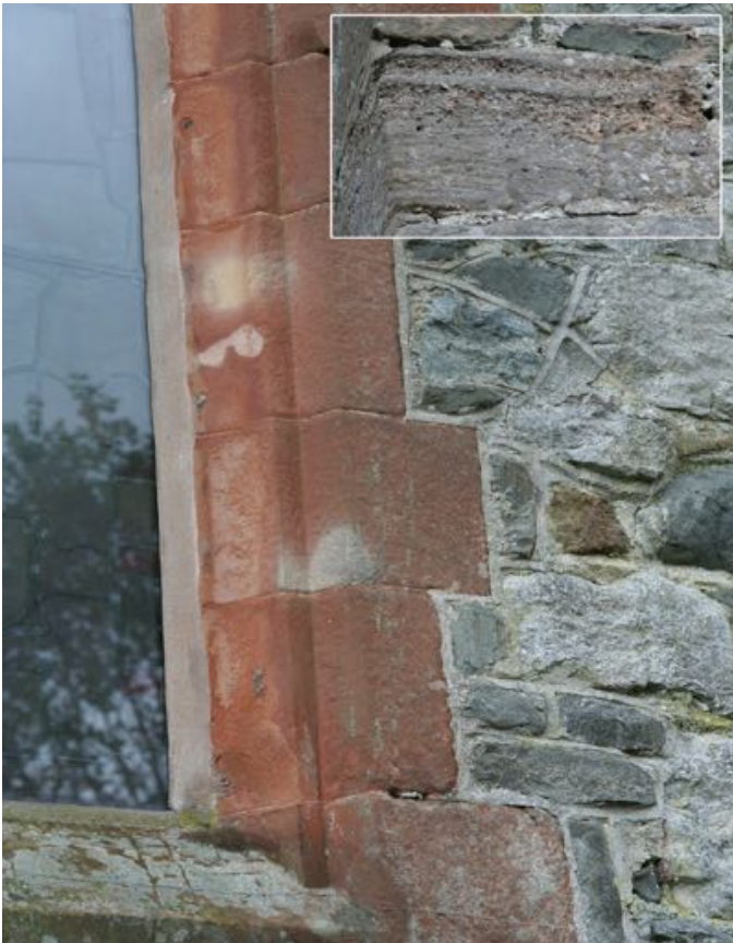
Fig. 1. (top left). St Ffraid's, Llansantffraid. Pale 'Old' Grinshill Sandstone dressing in window arch, rubble work including local Silurian (dark grey), red Grinshill / Ruyton and Westphalian age Salop / Etruria Formation (dark brown). Inset: 'new' Grinshill replacement. Fig. 2. (bottom left). Mottled Ruyton / Grinshill Stone, east window - St Ffraid's, Llansantffraid. Inset: details of pebbly (Grinshill Sandstone?) quoin. Fig. 3. (top right). West end of tower at St Tysilio & St Mary's Church, Meifod. Inset: detail of Grinshill quoins on south side. Fig. 4. (bottom right). Carved Celtic stone at St Tysilio & St Mary's Church, Meifod.
