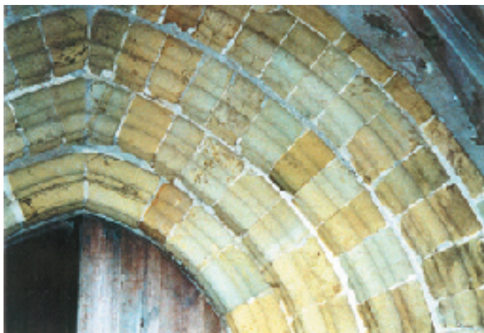
The church door (13th C) at Llanaber, north of Barmouth, showing some of the variation in colour and texture seen in the Egryn Stone.
