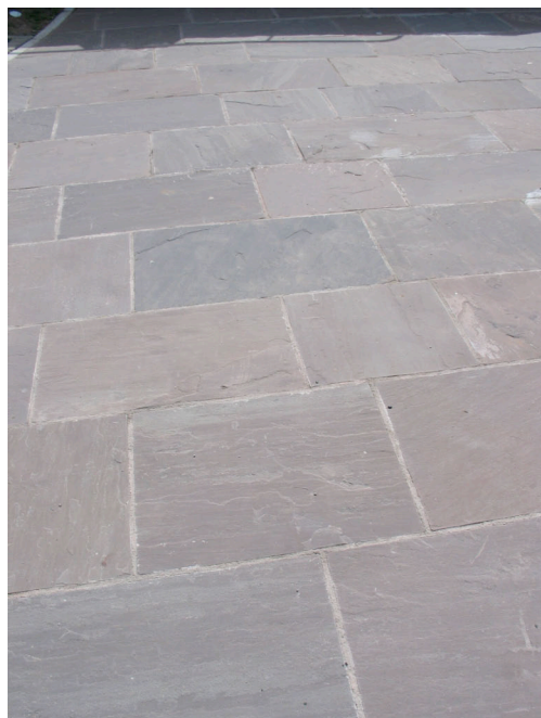
Fig.1. New locally produced ORS paving from the Black Mountains at the recently restored Old Monnow Bridge, Monmouth
