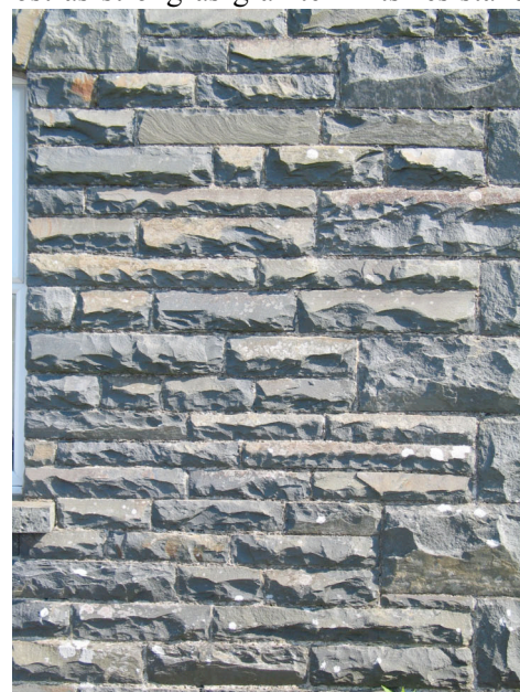
Fig 3. Close up of Llandewibrefi Bluestone rock-dressed facing.
