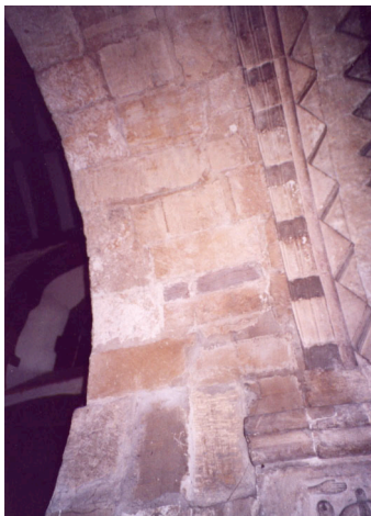
Fig 3. Detail of the arch, Beer Stone (?) and oolite mix
