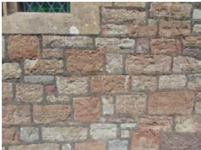
Fig. 1. Dressed Carboniferous Limestone, Pendoylan (©John Davies).
