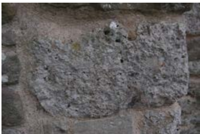
Fig. 1 (top) Banded sandstone in a fireplace, Usk Castle (©John Shipton). Fig. 2 (top right) Replacement sandstones in door jamb, possibly Red Wilderness Stone, Usk Castle (©John Shipton). Fig. 3 (bottom left) Tufa block in the wall of St Madoc's Church (©John Shipton). Fig. 4 (top opposite page) Large slabs of St Maughan's sandstone, St Madoc's Church (©John Shipton).
