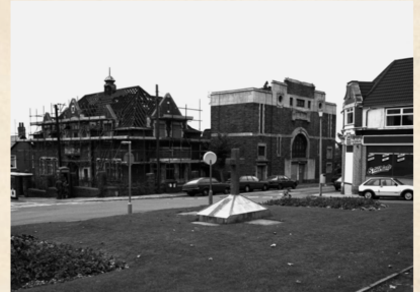
Y Stiwt ar hanner y gwaith datgymalu. The Institute being dismantled.
