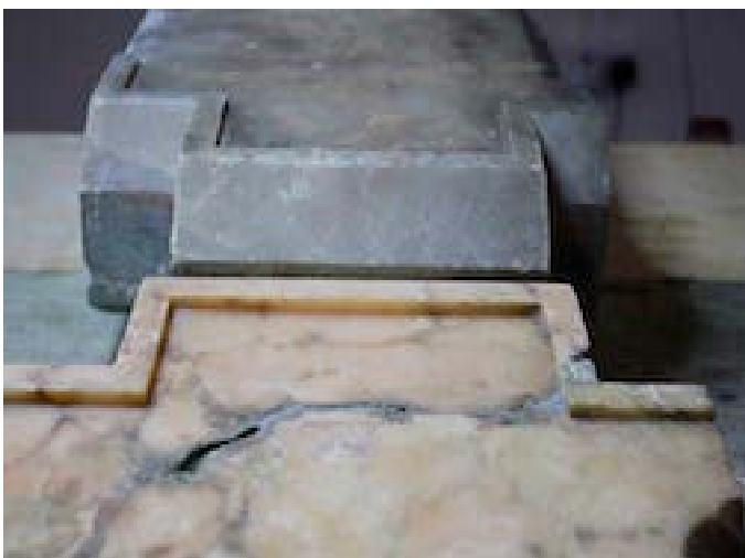
Fig. 5. (left) Chicken-wire Gypsum visible on the cleaned block in the foreground. ©Elliott Ryder Conservation.
