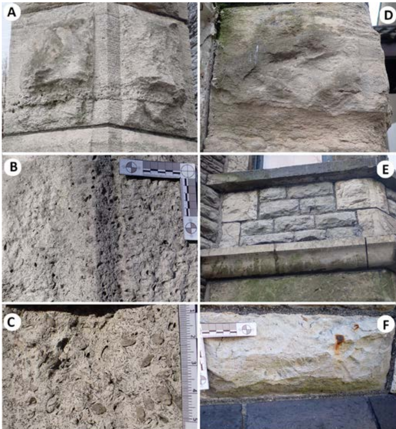
Fig. 6. Purbeck limestones at 135 Clive Road. A, mullion showing banding and a dense bed of Neomiodon . B/C, details of the mullion stone in A. D, quoin showing bedding and weathering. E, decorative course of Liassic limestone between ground and first floors. F, a block of Liassic limestone in the plinth.
