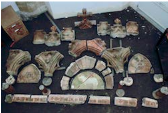
Fig. 1. (top left). The reredos in St Anne's church prior to dismantling. ©Elliott Ryder Conservation. Fig. 2. (bottom left). The dismantled upper section of the reredos. ©Elliott Ryder Conservation. Fig. 3. (top right) New stainless-steel restraint-fixings securing the reredos back to the brick wall. ©Elliott Ryder Conservation. Fig. 4. (bottom right). The core of the reredos built into the damp building fabric. ©Elliott Ryder Conservation.
