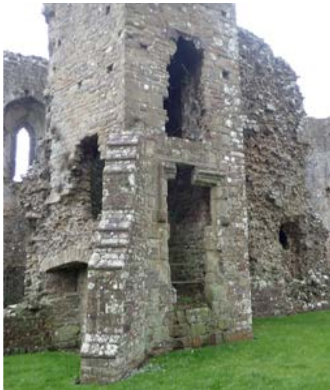
Fig. 7. South range of the castle, Cethings Sandstone blocks and dressings, with the exception of the second storey window, where there is a lintel of purple/red Caerbwdy Sandstone.
