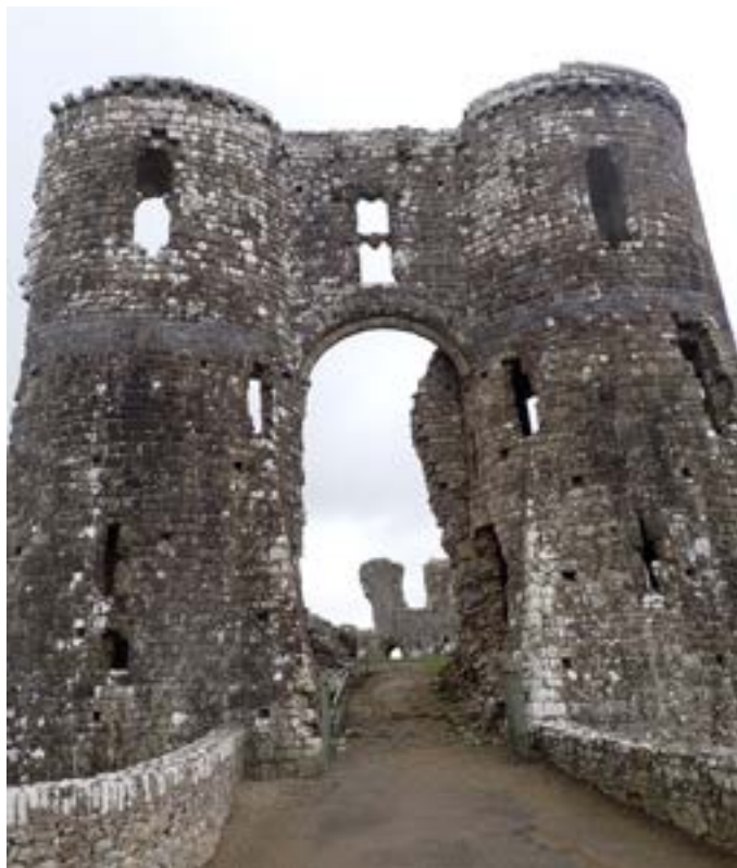
Fig. 6. Llawhaden Castle gatehouse worked from squarred Cethings Sandstone blocks, with a frieze of black Carboniferous Limestone.
