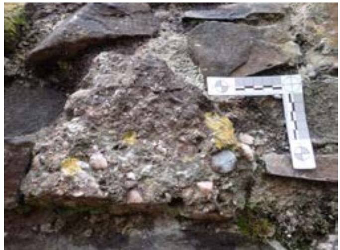
Fig.2. Conglomerate (Basal Conglomerate) associated with the Cethings Sandstone. Wiston Castle). Scale bar in cm.
