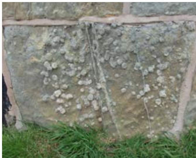
Fig X. A block of the Esk Bed with barytes nodules.
