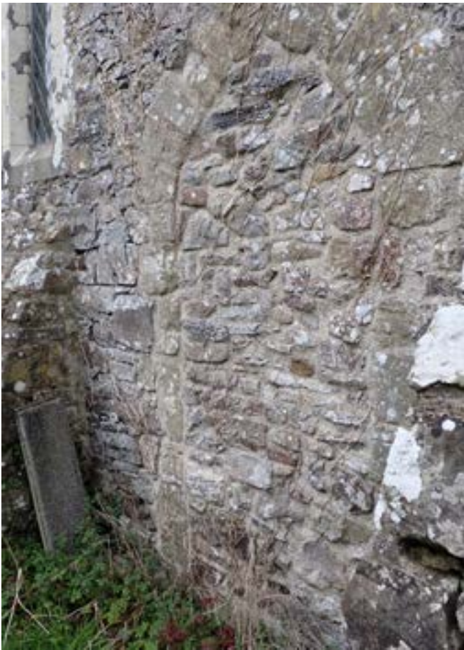
Fig. 5. St Marys Magdelen, Wiston. Fabric of rubble Carboniferous Limestones and block doorway dressing of buff Cethings Sandstone.
