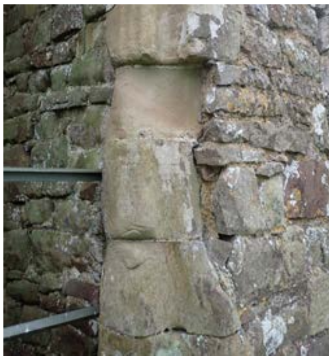
Fig. 8. Close up of Cethings Sandstone doorway dressing in Fig. 7.
