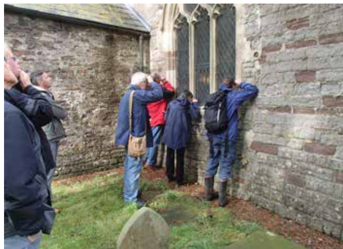
Figure 2. St Bridget's church, St Brides. South wall to the east of the porch, of coursed Liassic limestone blocks and Triassic sandstone. Photo Graham Oliver.
