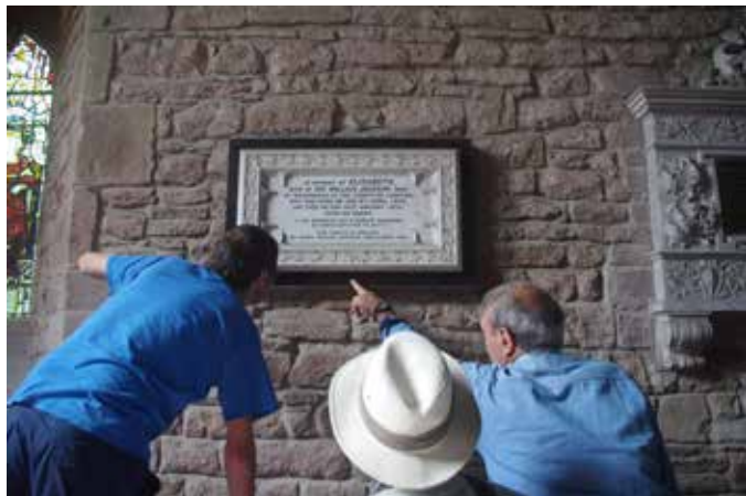
Figure 5. Carrara Marble memorial plaque on a possible Cornish serpentine backing.
