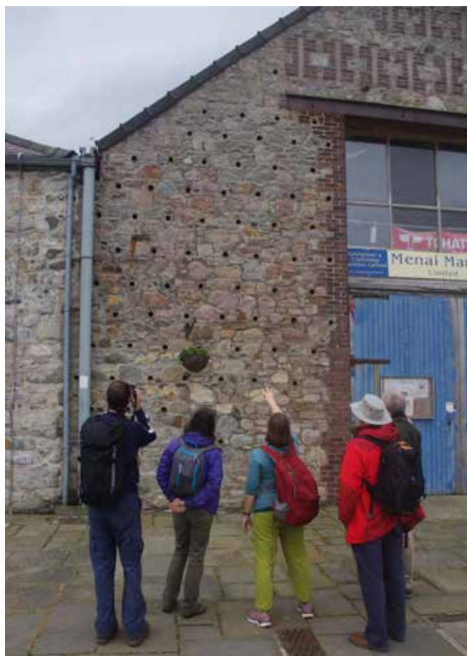
Figure 8. Warehouse with clay pipes inset in to rubble walls, Caernarfon.
