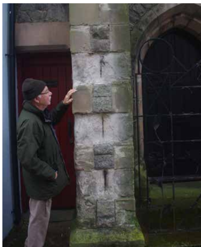
Figure 10. Masonic Lodge Chapel with badly weathered columns and buttresses.
