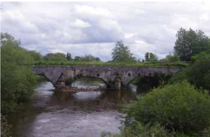
Figure 2. Aqueduct over the River Vyrnwy, probably built of Cefn Sandstone.
