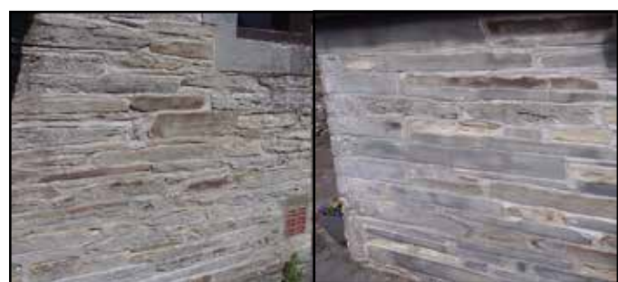
Figure 2. Old fabric left, new sawn blocks, right.
