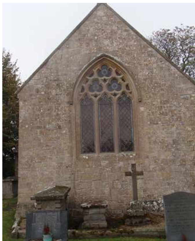
Figure 3. East elevation of St Mary Magdalene church, Goldcliff showing cut blocks of pale limestone. Photo Graham Oliver.
